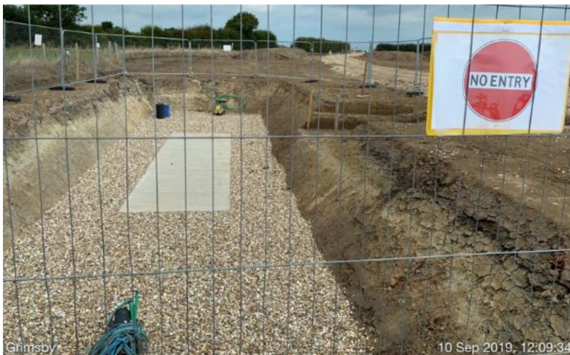
Figure 47 Example image of a concrete slab in the base of an excavated joint bay (Source - Grimsby, Hornsea 2 Offshore Wind Farm)
