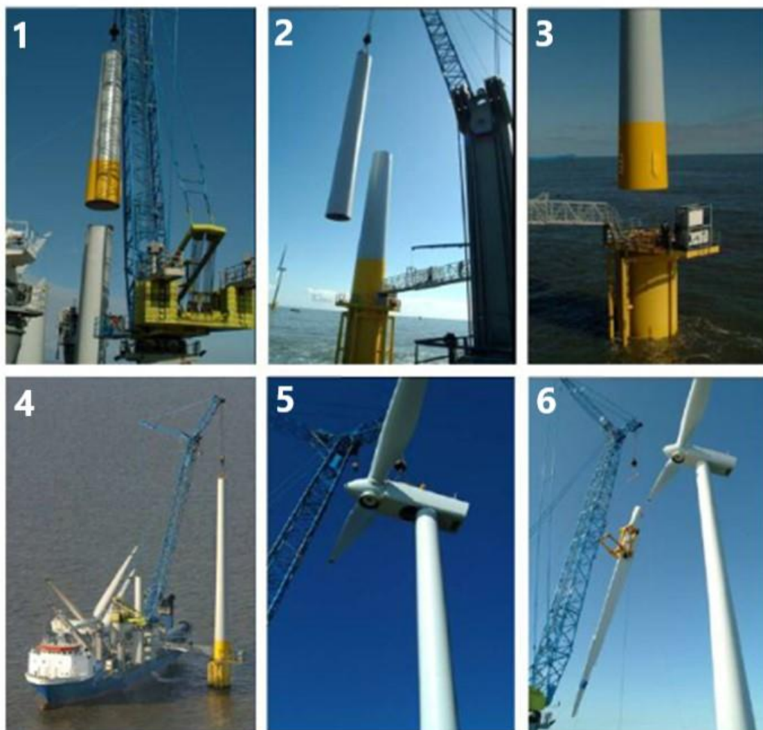
Figure 22 Sequential photographs of installation of turbine tower, nacelle and blades
