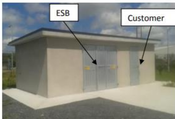
Figure 101 Freestanding MV substation adjoining a customer's switch room (Source ESB Networks Construction Standards for MV Substation Buildings)
