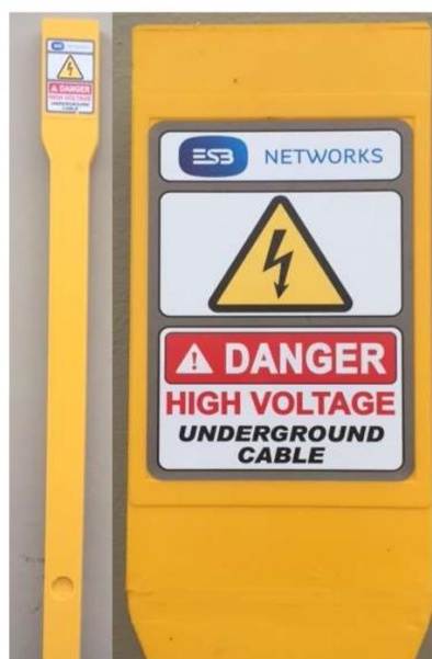
Figure 53 Typical HV cable marker post
