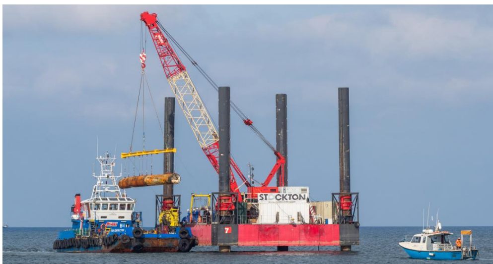
Figure 38 Example image of MTBM recovery of steel pipe and drill head from seabed (Source Stockton Drilling)
