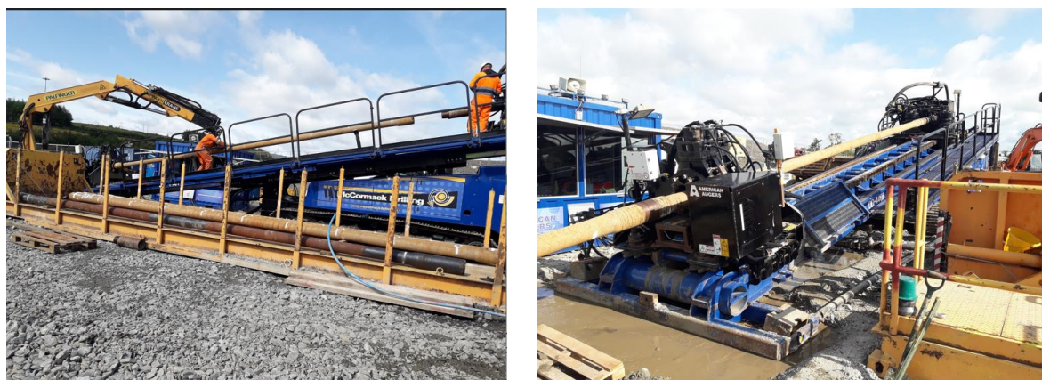
Figure 64 Example image of a typical HDD Rig set up (DD-440T) (Source J. Murphy & Sons Limited)
