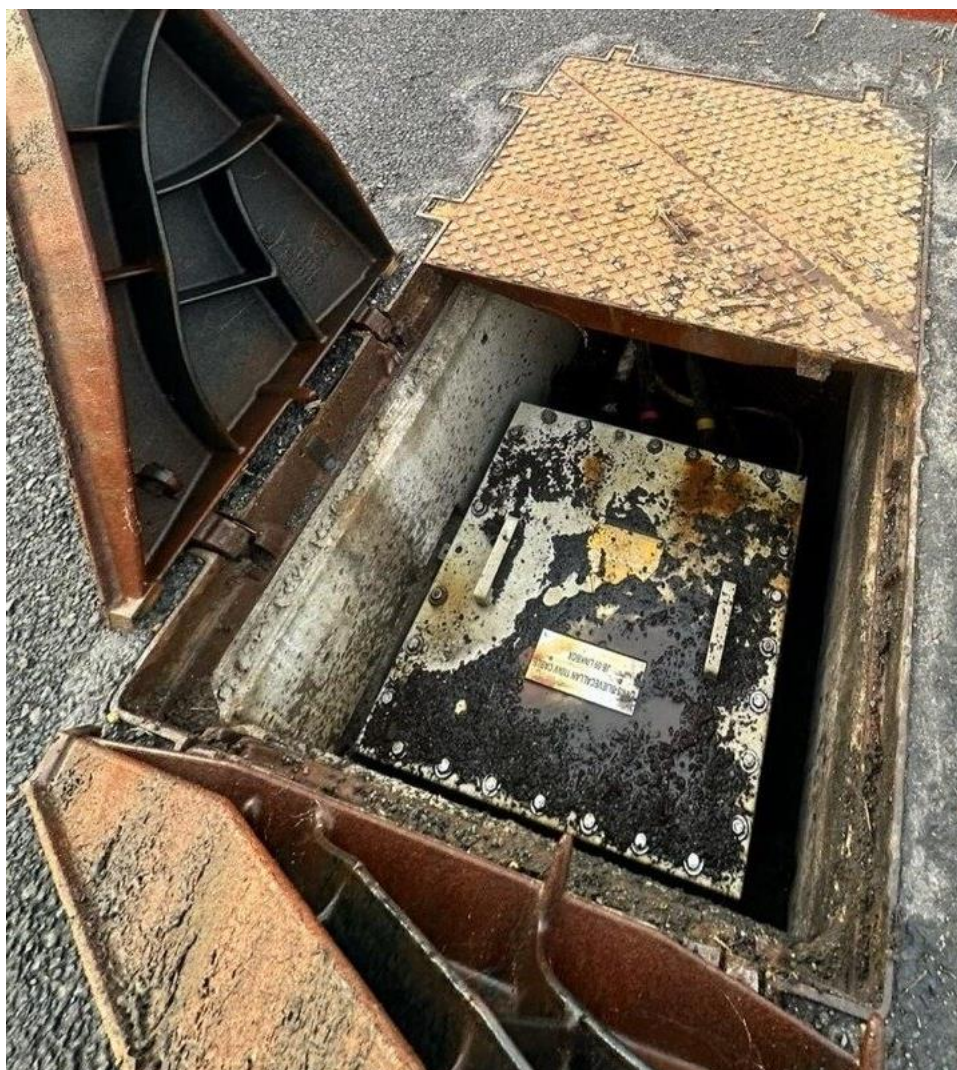
Figure 49 Example of an open Link Box Chamber Inspection cover
