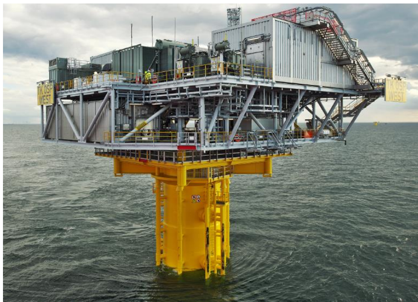
Figure 13 An example of an offshore substation platform on monopile foundation, Triton Knoll Offshore Wind Farm (RWE).
