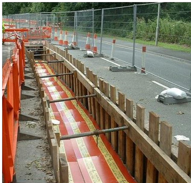
Figure 67 Example image of open cut trench in public road supported by trench box
