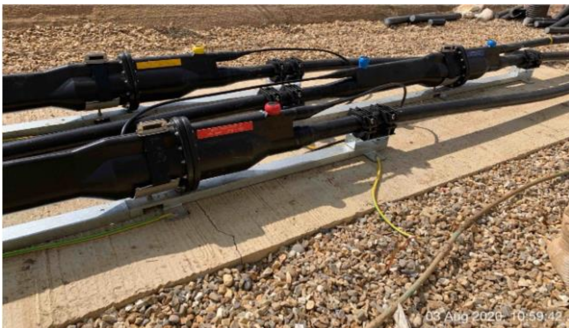
Figure 39 Export cable joints laid over the concrete plinth of a TJB (Source - Grimsby, Hornsea 2 Offshore Wind Farm)
