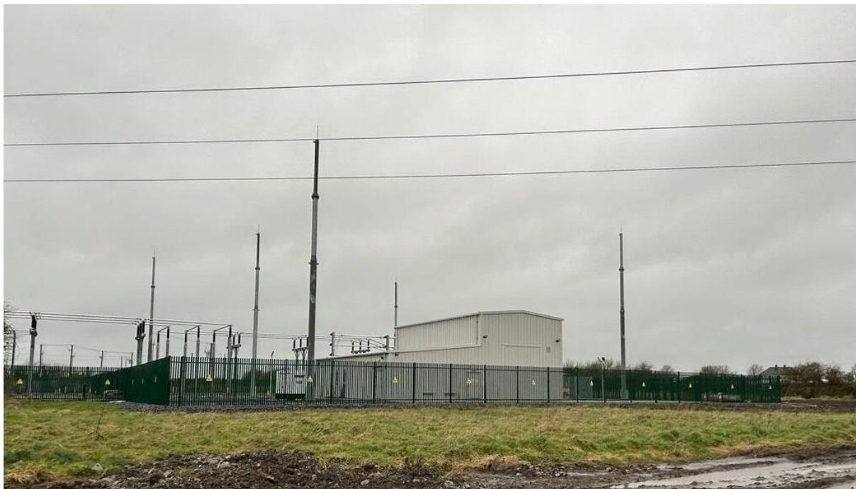
Figure 78 Example image of a Statcom building with lightning protection
