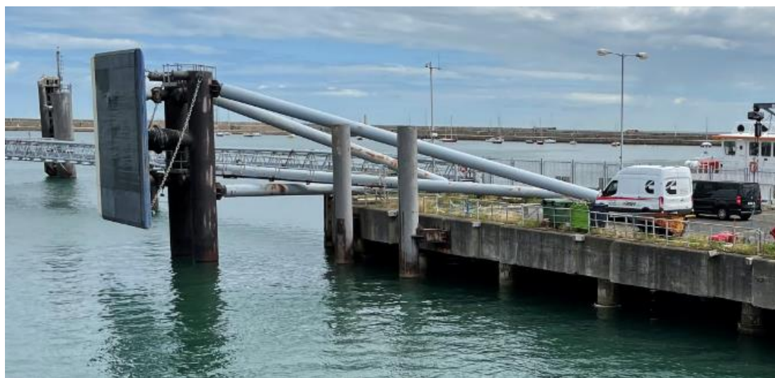
Figure 86 Existing fender structure and supporting steelwork at St. Michael's Pier
