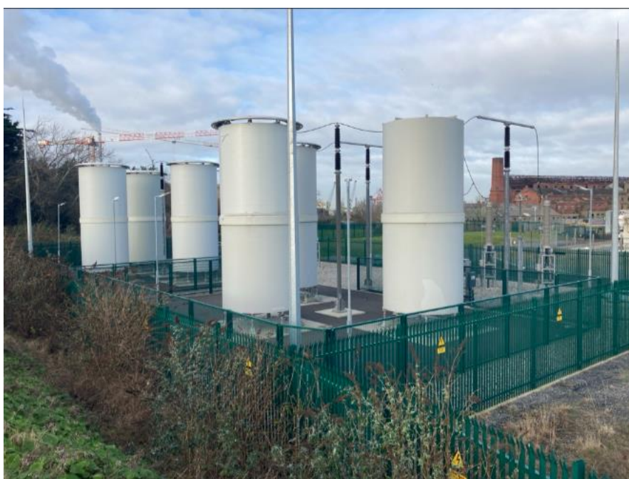
Figure 72 Example image of shunt reactors in an onshore substation compound, with lightning protection
