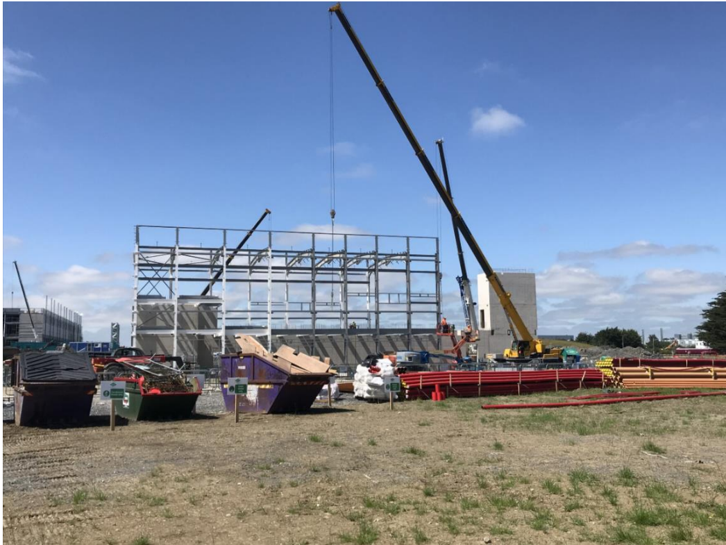
Figure 74 Example image of a GIS building steel frame under construction
